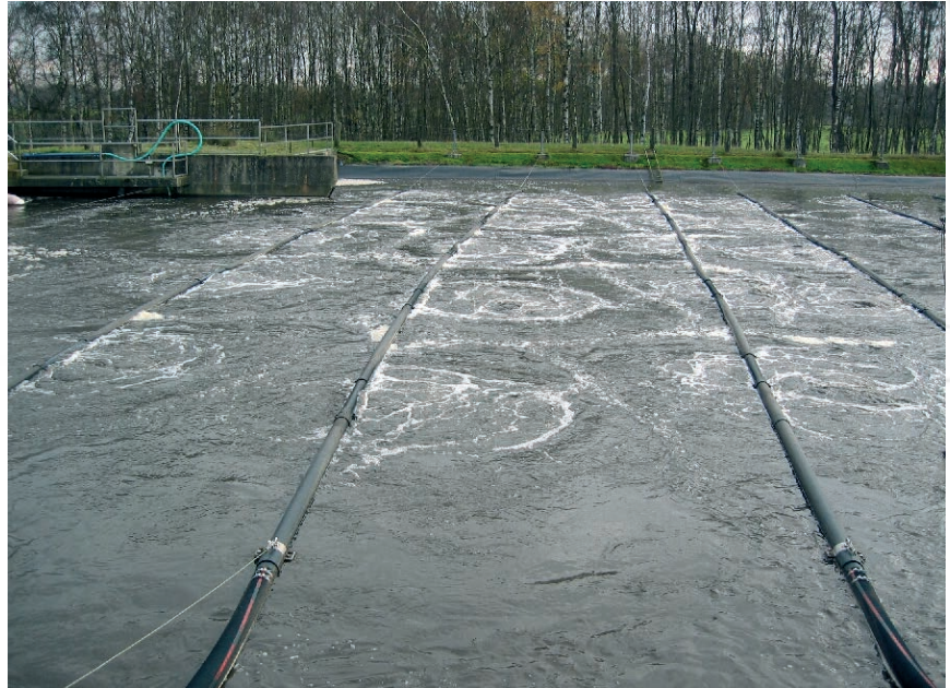
E-FLEX ® -FLOAT -Aeration Chains in an activated sludge tank
