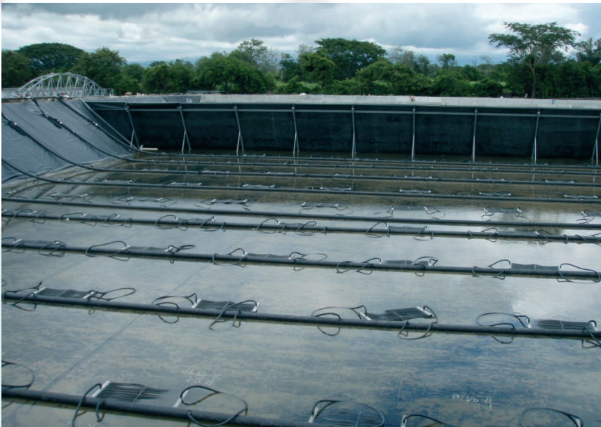
E-FLEX ® -FLOAT-Aeration Chains in a lagoon-type activated sludge tank
