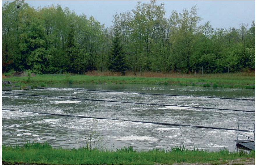
E-FLEX ® -FLOAT-Aeration System in an aerated lagoon
