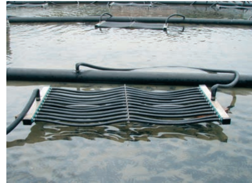
E-FLEX ® -FLOAT-Aeration System before start-up
