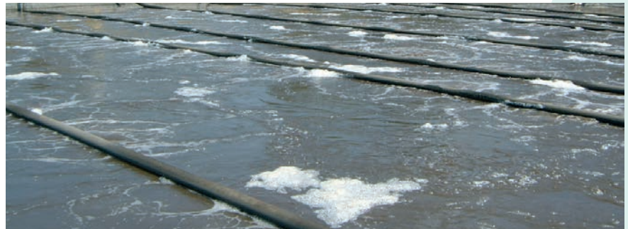
E-FLEX ® -FLOAT -Aeration Chains in an activated sludge tank
