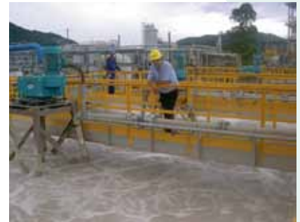
5 HYPERCLASSIC® -Mixing & Aeration Systems in an industrial wwtpt in Brazil (Chemical Industry)
