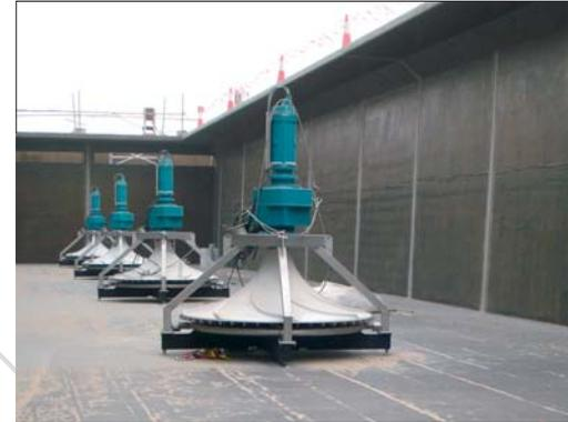
**HYPERDIVE®** Mixing & Aeration System during installation in a municipal wwtp in Middle East
