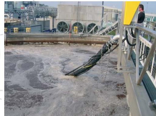
**HYPERDIVE®** Mixing & Aeration System in operation in an industrial wwtp in Sweden (Pulp & Paper Industry)
