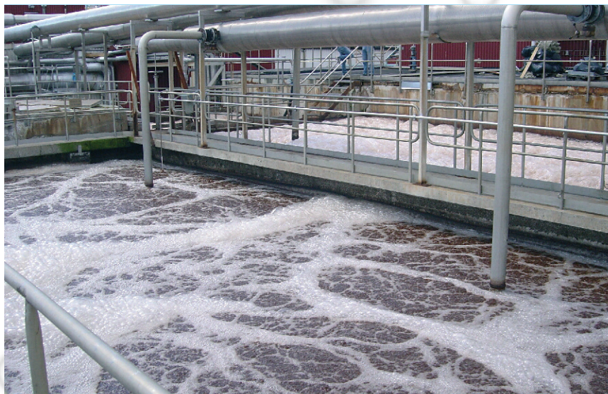
TEX-FLEX aeration system in an industrial wastewater treatment plant in Sweden (Pulp & Paper Industry)
