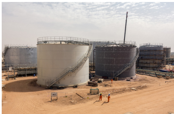
Drinking water reservoir in steel construction
