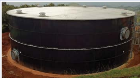
Trough Deck Roof
